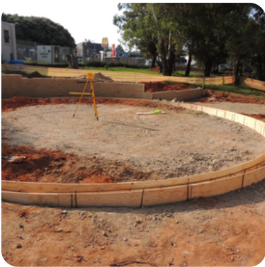
Our Water Storage Tanks team checked the levels and prepared the grounds for assembling our 3 Water Storage Tanks.
