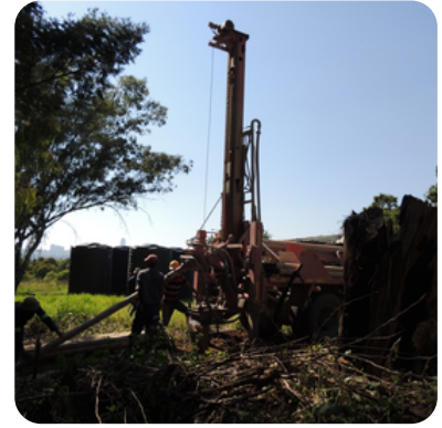
We drilled a new 51 meters borehole across the dirt road from the Water Treatment Plant.
