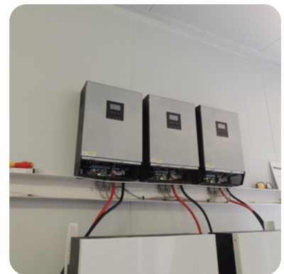
We installed a power back up system to ensure a continuous feed of water to the College when there is load shedding or no electricity in the College.
