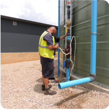
Our technicians completed the installation of water meters, flowmeters, pressure gauges and automating the water system.
