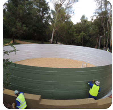
We completed assembling the 545 000L water tank and began with the 60 000L water tank which was completed in the same week.
