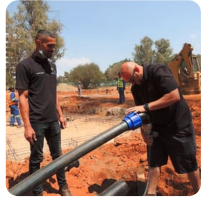
Our technicians came to complete a successful pressure check on the entire water pipeline and found no leaks at the joints.
