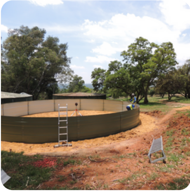
We commenced the assembling of the 270 000L Water Storage Tanks.
