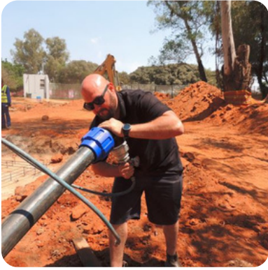
Our technicians came to complete a successful pressure check on the entire water pipeline and found no leaks at the joints.
