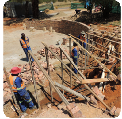
We continued building the retaining walls for the water tanks and leveling the foundation of the building.
