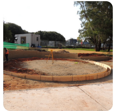
Our Water Storage Tanks team checked the levels and prepared the grounds for assembling our 3 Water Storage Tanks.
