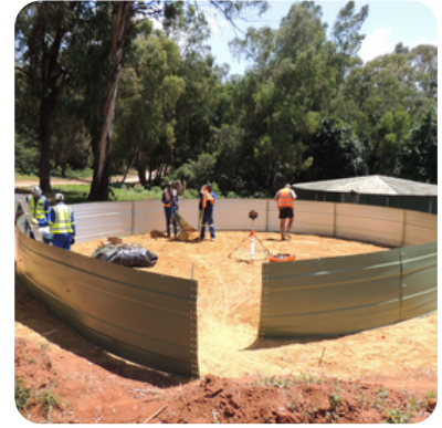
We commenced the assembling of the 270 000L Water Storage Tanks.
