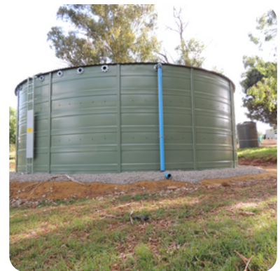
We completed assembling our 270 000L water tank and began assembling the housing unit.
