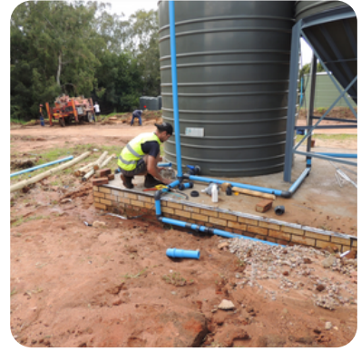
Our technicians completed the installation of water meters, flowmeters, pressure gauges and automating the water system.
