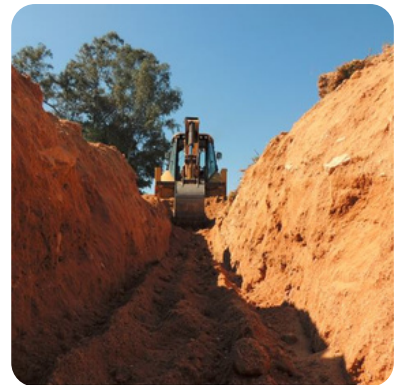
We commenced digging trenches at Higher Ground, inserting water pipes and closing the trenches within a couple of days.
