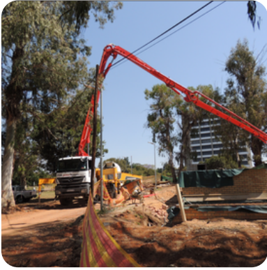
We completed the pouring of the concrete slabs on Thursday 21st October.
