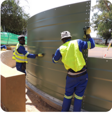
We completed assembling the 545 000L water tank and began with the 60 000L water tank which was completed in the same week.
