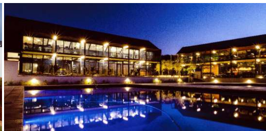
5ive on Thirteenth Luxury Apartments Wayne: 072 139 4415
